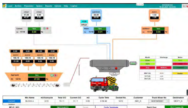
Control System & AQ-SMART Software
